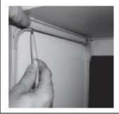
Mark the distance between fittings and cut off the measured length of the horizontal guide.
