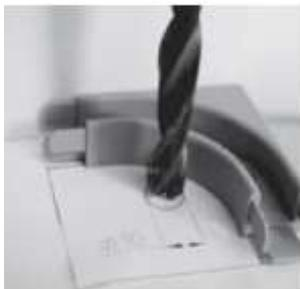
In the spot marked on the template, with  $\varnothing 10$  drill drill hole depth 11-12 mm.
