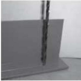
In the end strip drill a holes for fixing screws.
